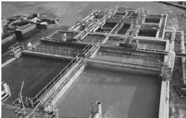
**Figure 31.** Wheal Jane HDS plant showing the reactors and lamella clarifiers
