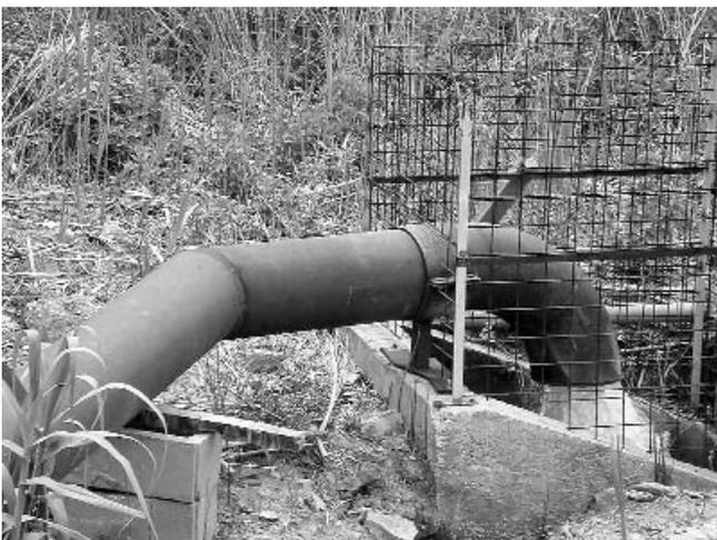
**Figure 23.** Water pumping system at the Gavorrano underground mine (at present, about 80 L/s)
