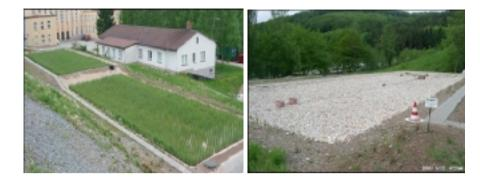
Figure 10. Experimental multi-cell wetland at WISMUT's Schlema mine site (left: plant cells, right: microbiological cell with gravel bed)
