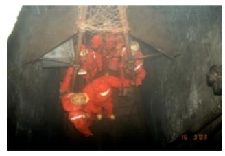
Figure 15: Rescue of miners with safety winch
