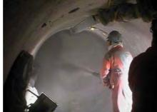
Figure 8: Example of shotcrete plug at Febex experiment [7]
