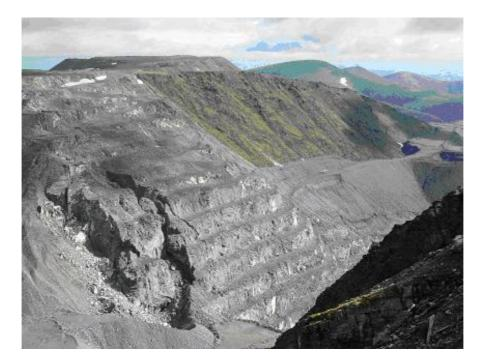
Figure 4 West-North pit wall of Tsentralny mine failure
