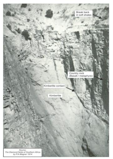
*Figure 4* Kimberlite pipe showing clear contact between pipe and country rock (Kimberley Mine) Wagner 1914
