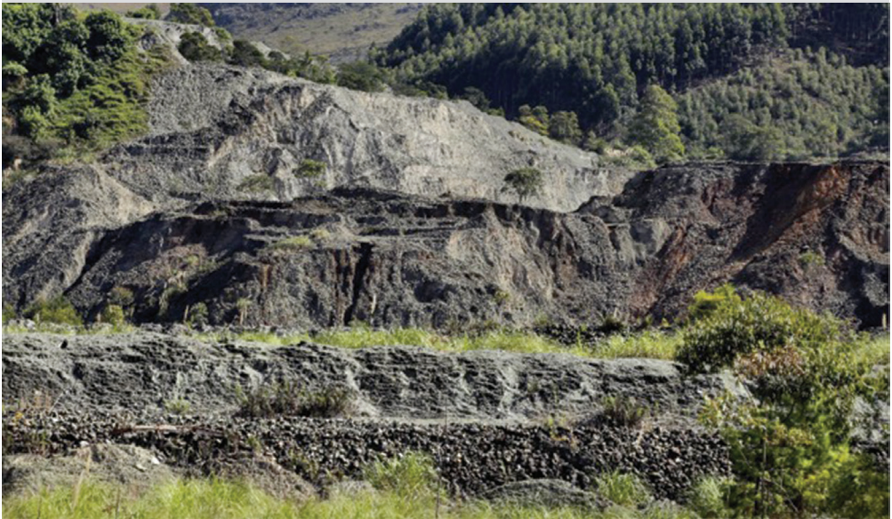
Figure 2 Largely unremediated asbestos tailings and waste rock at the former Havelock asbestos mine, eSwatini
